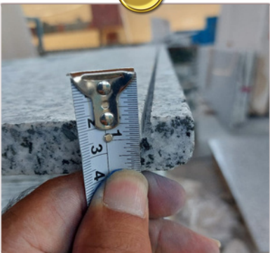
Water dripline / Groove
